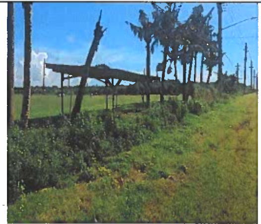
Figure 4 - Standing along Route 15, this temporary structure marks a corner of the 200' access and utilities R/W (Lot 3R/W)
